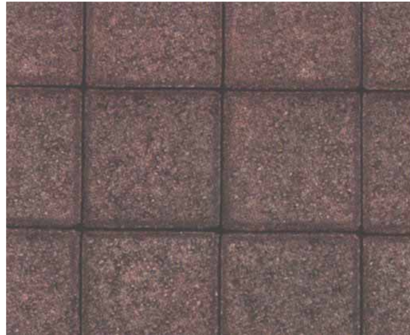
Figure 4.3 Special Pedestrian Paving #2 - Concrete Unit Pavers
